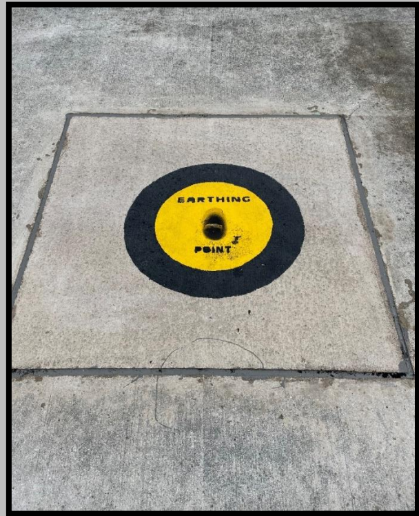
Completed earthing point
