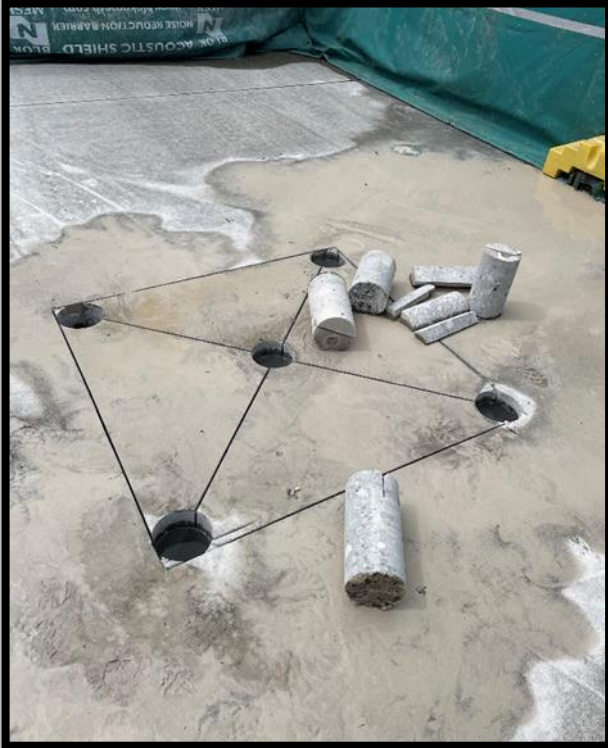
Core-drilling for earthing receptacles
