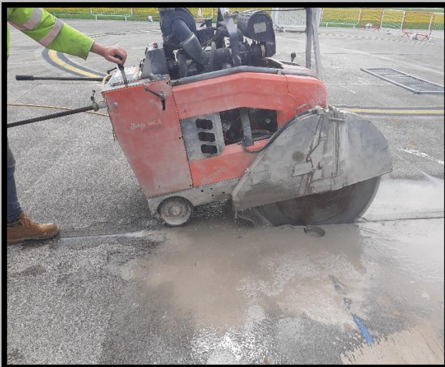
Saw cutting concrete
