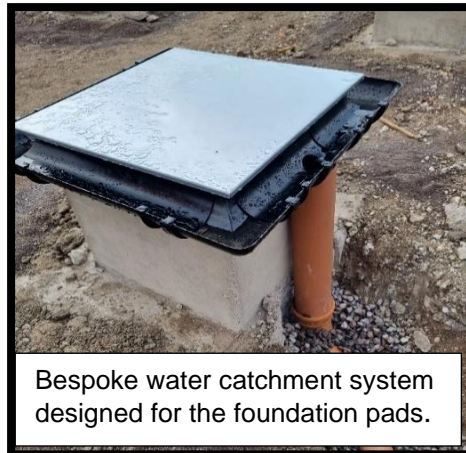
Cast Concrete Foundation Pads, Ready to Accept Modular Units
