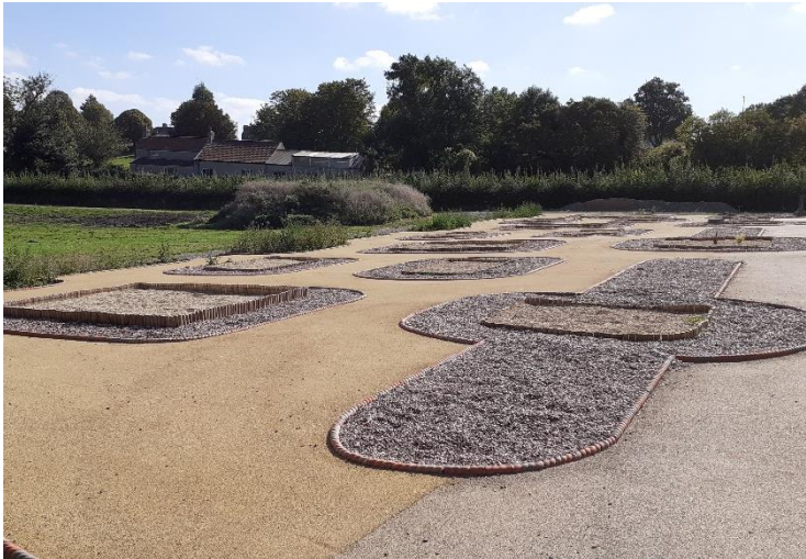
Supply, lay and compact Type 1, 20mm asphalt base course and topped with Tarmac Ulti-Colour®
