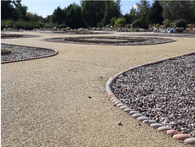
Supply, lay and compact Type 1, 20mm asphalt base course and topped with Tarmac Ulti-Colour®
