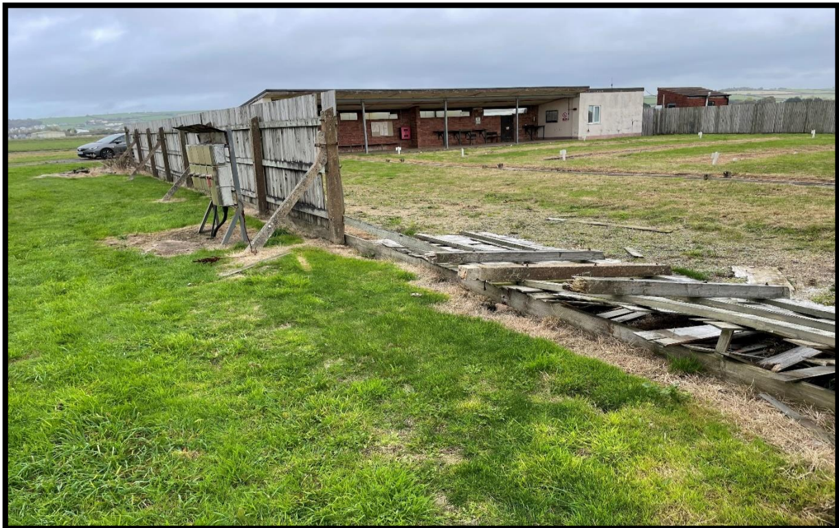
Existing Fence Line RMB Chivenor
